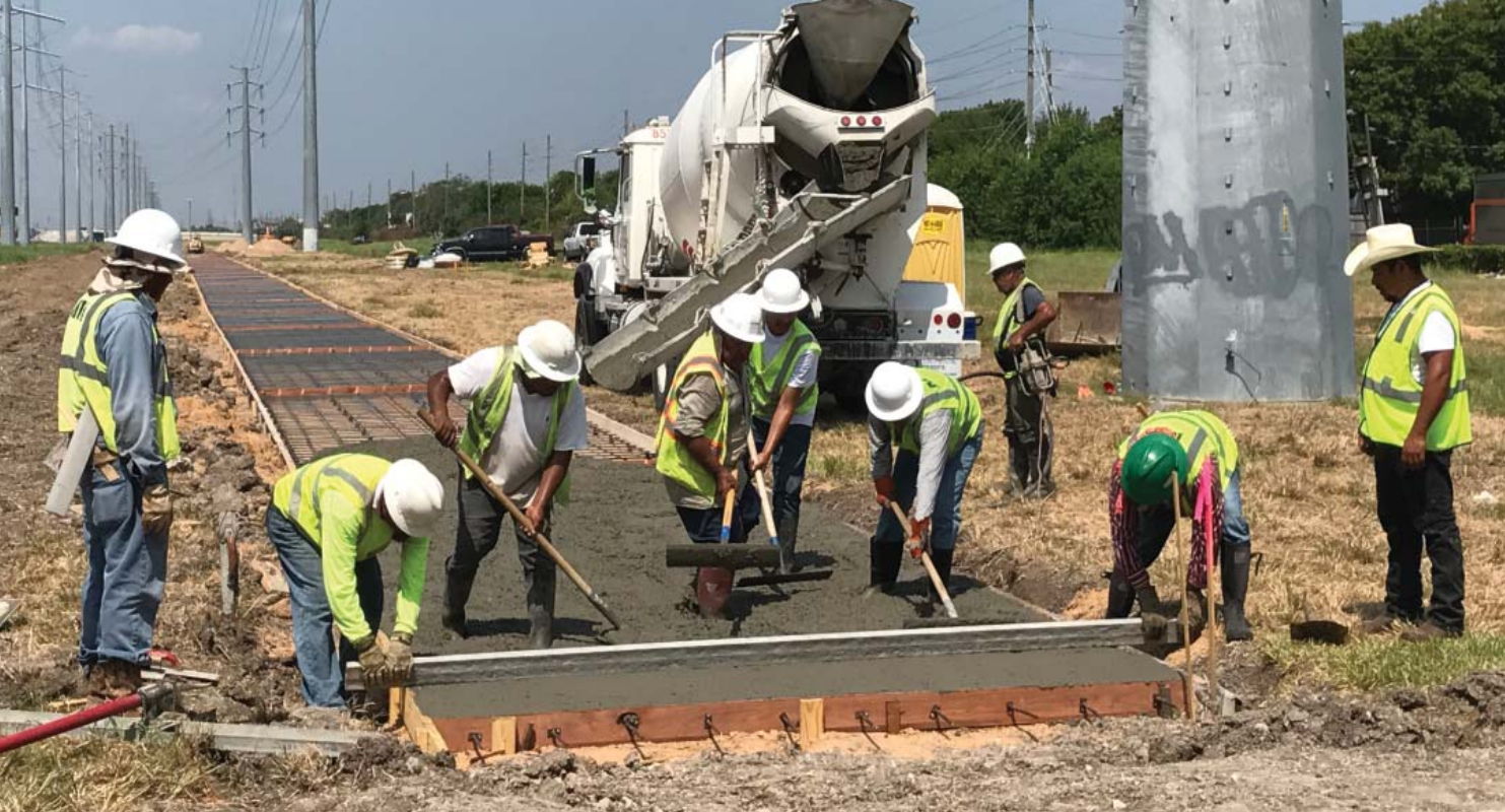
Pour Me Another: In August, workers began pouring concrete for the latest addition to the Westchase District trail system, the Westpark Trail. This 10-foot-wide trail is located just north of the Westpark Tollway, runs .6 miles east-west between South Gessner Road and Briarpark Drive, and connects to METRO’s Gessner Park & Ride lot.
